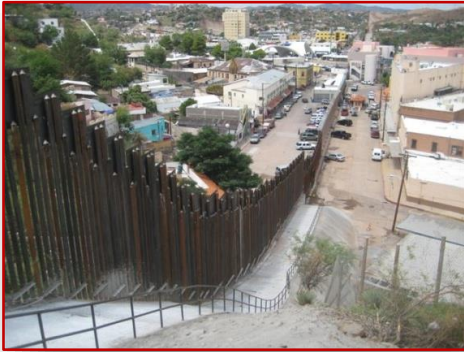
Nogales, Ariz., Border Fence Replacement
